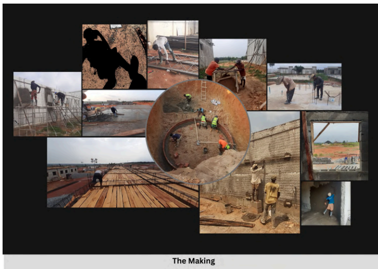
Figure 2. The Making. Eleven photographs of workers laying blocks with hand-mixed mortar, screeding a slab on timber formwork, tying reinforcement steel by hand, and excavating a soakaway pit manually. Photo Credit: Author.
