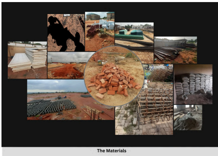
Figure 1. The Materials. Eleven photographs taken between December 2025 and March 2026, showing sandcrete blocks in pre-laid rows, loose laterite bricks, steel rods, cement bags, and roofing sheets. The arrangement of the blocks reflects construction-sequence decisions made by workers. Photo Credit: Author.
